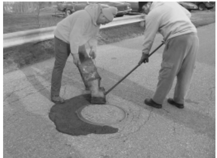
Spreading material around a manhole with a rectangular trough lute.
